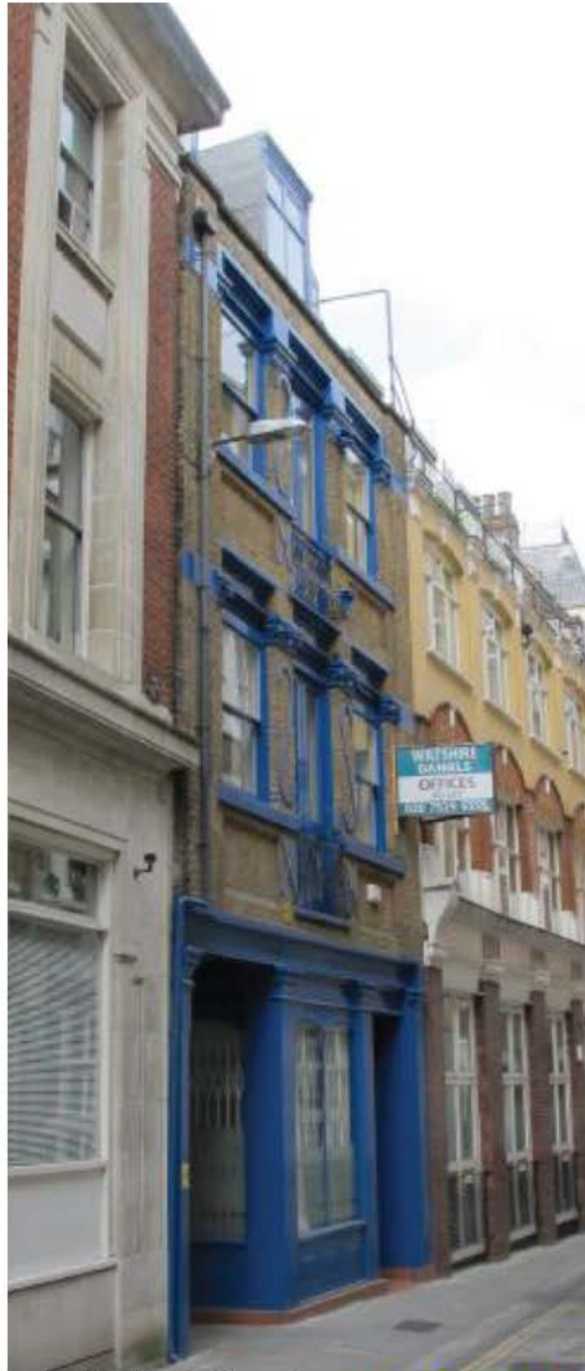
75 Carter Lane: View from Carter Lane looking west
